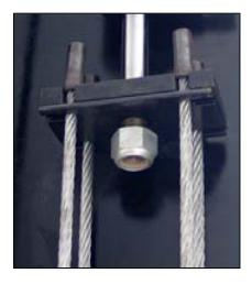
6. Locate the four cable ends and route the appropriate Cable through each hole in corners of the Mainside Runway, shown in Figure # 4. Take up as much cable slack as possible and lay each cable back into the runway. <u>Note:</u> Make sure that cables are properly routed around pulleys and are not in a bind. Refer to Figure 4 for Cable routing detail.
