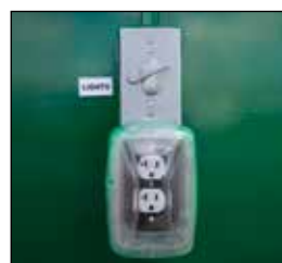
Weatherproof GFI receptacle and light switch
