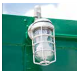
Vapor-resistant exterior light with photocell
